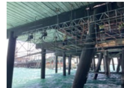
Scaffolding in place for Pile Wrapping Project
